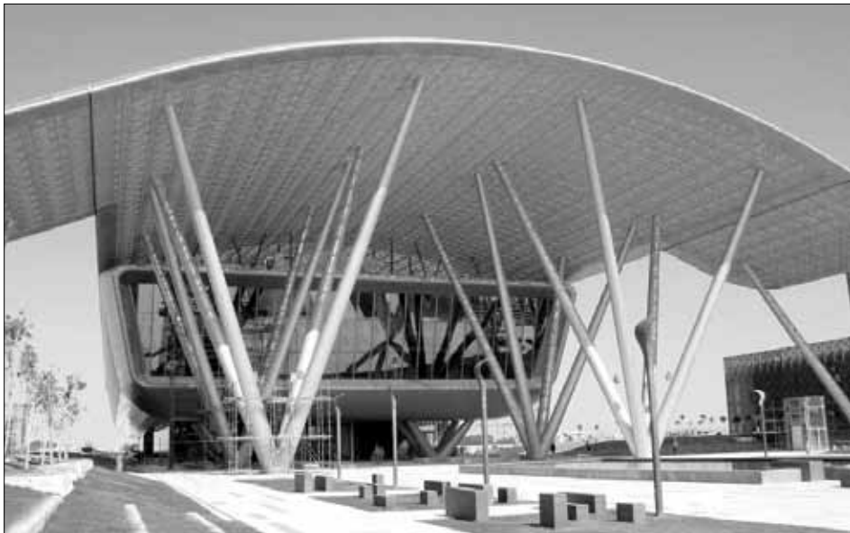
Figure 1.2.8: The striking Qatar Science & Technology Park (QSTP) designed by world-renowned architects Woods Bagot
