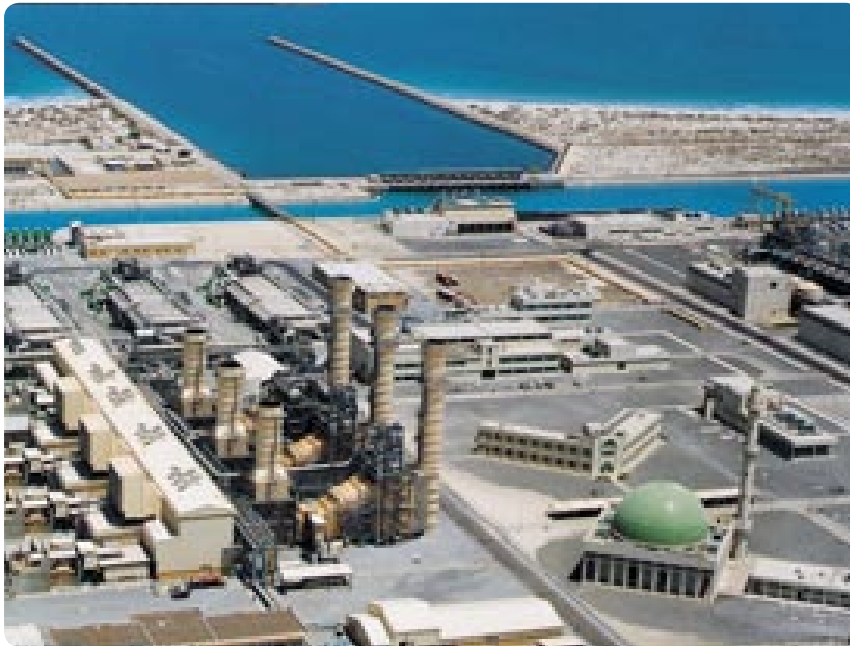
Al Taweelah Power Plant in Abu Dhabi, United Arab Emirates
